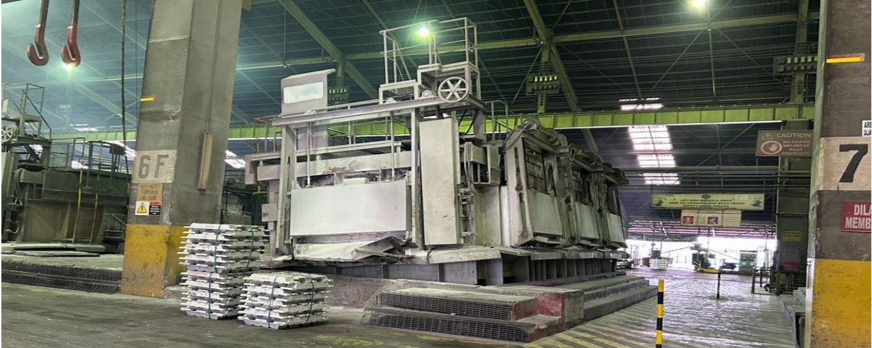
Figure 1 - The Aluminum casting plant in real world
